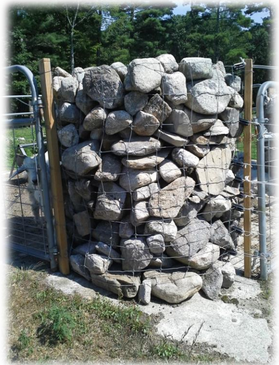
Up close photo showing fencing used to create a crib to hold the stones and wood posts to attach the gates
